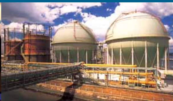
City Gas production facilities at Senoko Gasworks
